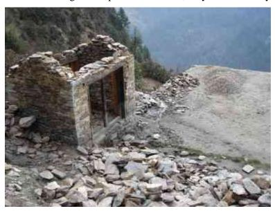
for the new toilet. According to the contractor, new cut stone will be used for the outside wall and stone from old toilet will be used for the inside the wall. They have a plan to go for the toilet construction as soon as interior decoration of the new building is completed.
