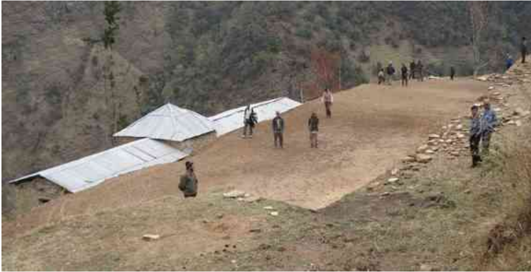
Ground for the Sagaramatha Primary School reconstruction Project
