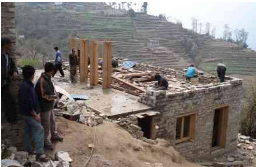
Science lab building is being constructed
