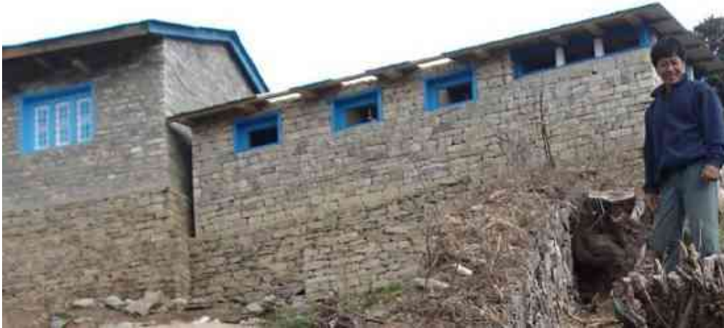
Sagar Bakanje School newly constructed toilet. View from down of the toilet
