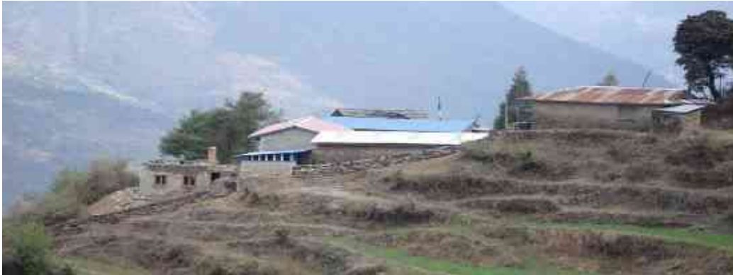
Bakanje School with new toilet and science lab are being constructed
