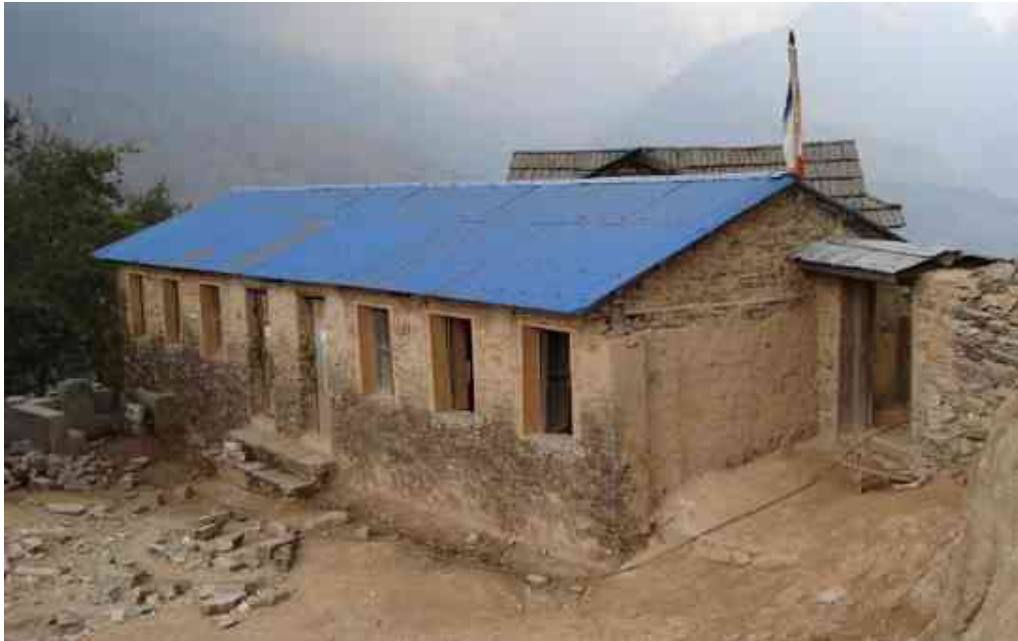
Earthquake resistance building after replaced the old windows with new.
