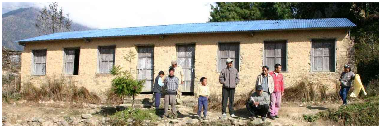
One of the Earthquake resistant School Houses
