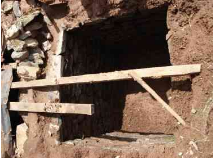
Septic tank of the toilet and sanitary complex is being constructed at Pikey Lower Secondary School, Tamakhani VDC
