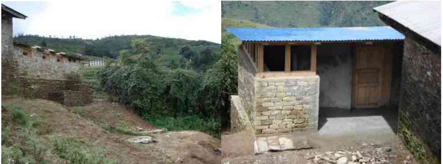
Newly- constructed Toilet & Sanitary Complex at Chandra Jyoti Lower Secondary School, Bakanje Solukhumbu
