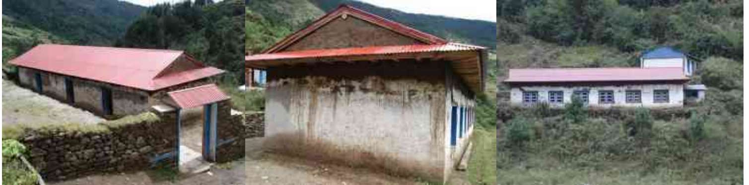
Completed Mopung Primary School Re-roofing Project, Beni VDC ward no. 5 Mopung, Solukhumbu
