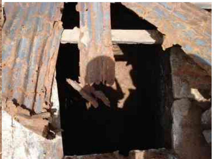
Septic tank of the toilet and sanitary complex is being constructed at Pikey Lower Secondary School, Tamakhani VDC
