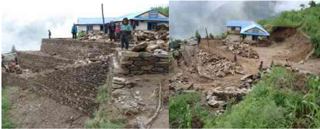
Chhimbu School playground under is under construction
