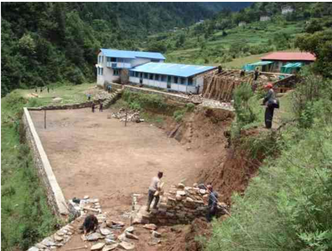
Stones stairs being constructed at Pikey Lower secondary School
