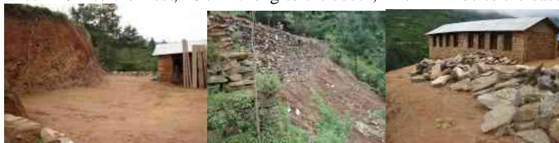
Tamakhani School playground is under construction
