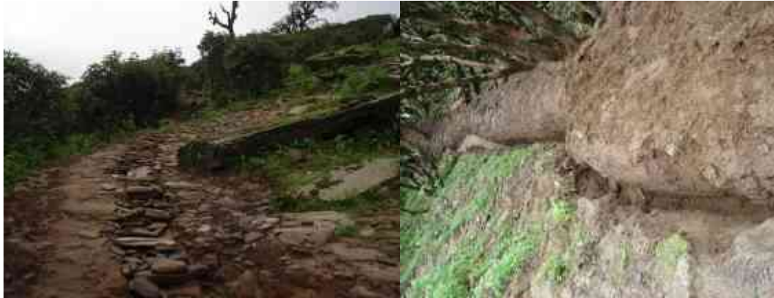
Lanjura Drinking Water supply Project is under Construction
