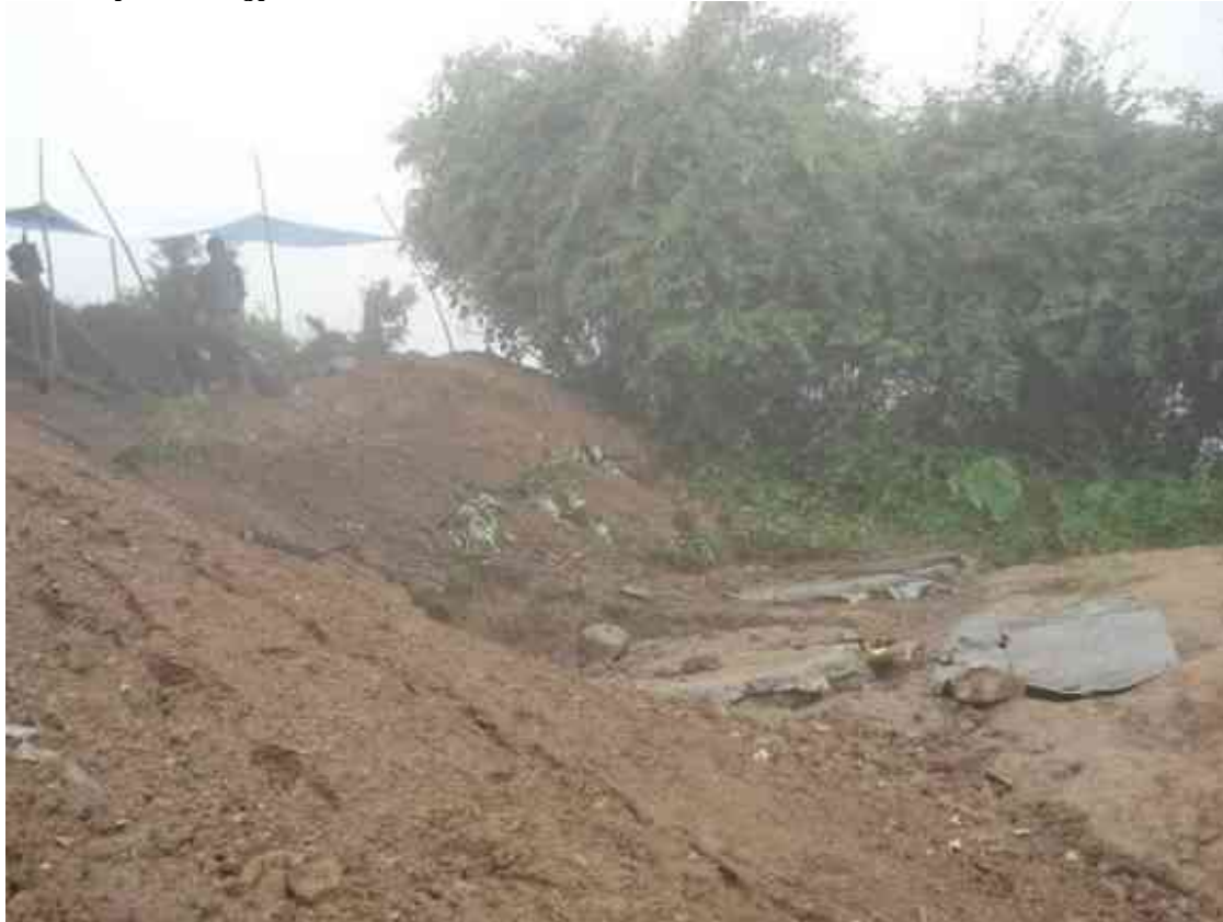
Sagar Bakanje toilet is under construction
