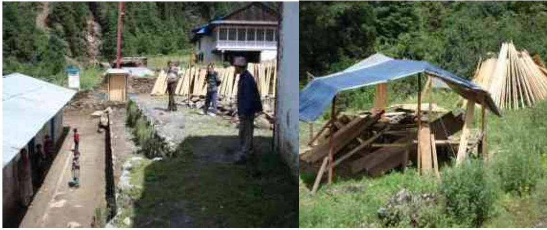
Mopung School Re-roofing work is being done
