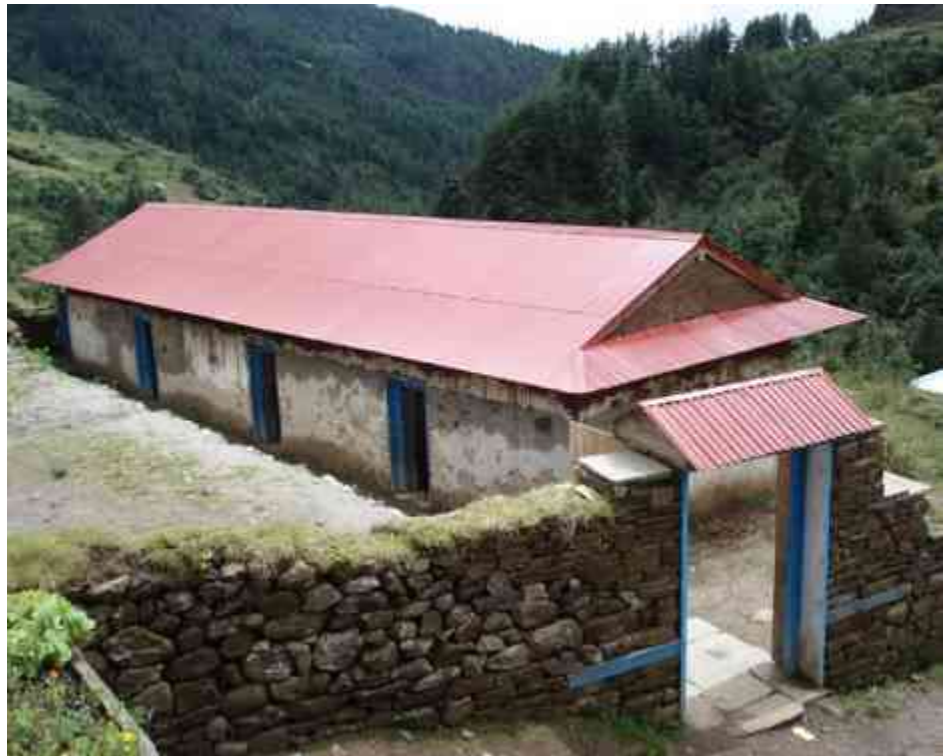
Mopung Primary School after completion of the re-roofing
