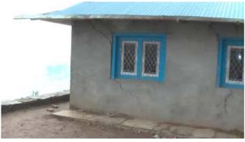
building was completed with cement plaster and roof. But then the summer monsoon period started with heavy rain fall, and soon big crags were seen in the cement surface. And by mid July the supporting wall and the house end fell down. Shortly after also his back wall of the playground fell down, and almost simultaneously the nursery wall fell.
