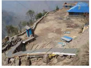
Cement topping on the wall at the roadside is underway. Topping on the one side wall has completed and it has got the thickness of 10 cm. Next side is yet to be started. As major contractor for the cement work Ang Gelu says that topping of the next wall will start immediately, for that cement and sand are ready. I havenøt found any comment about the cement plastering and cement topping sofar
